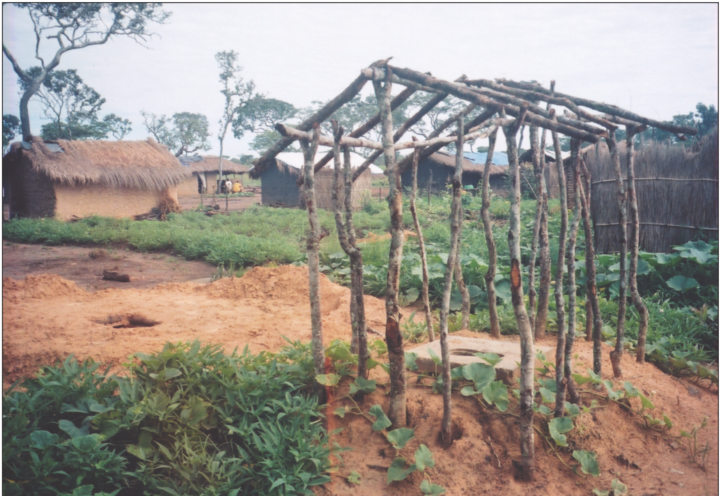
Family pit latrine under construction
