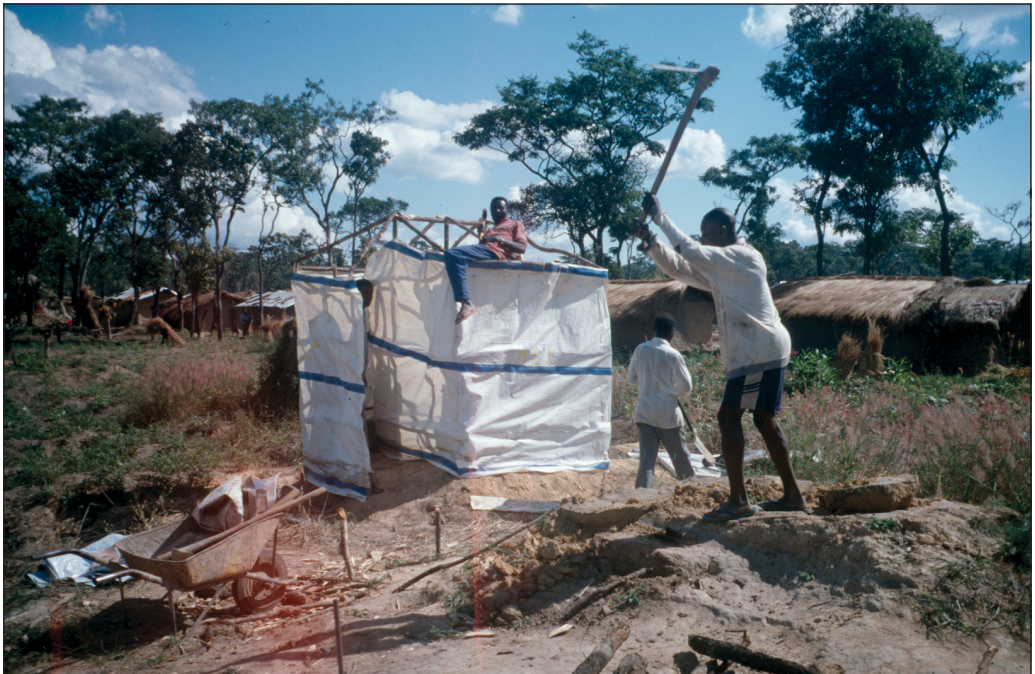
Pit latrine construction
