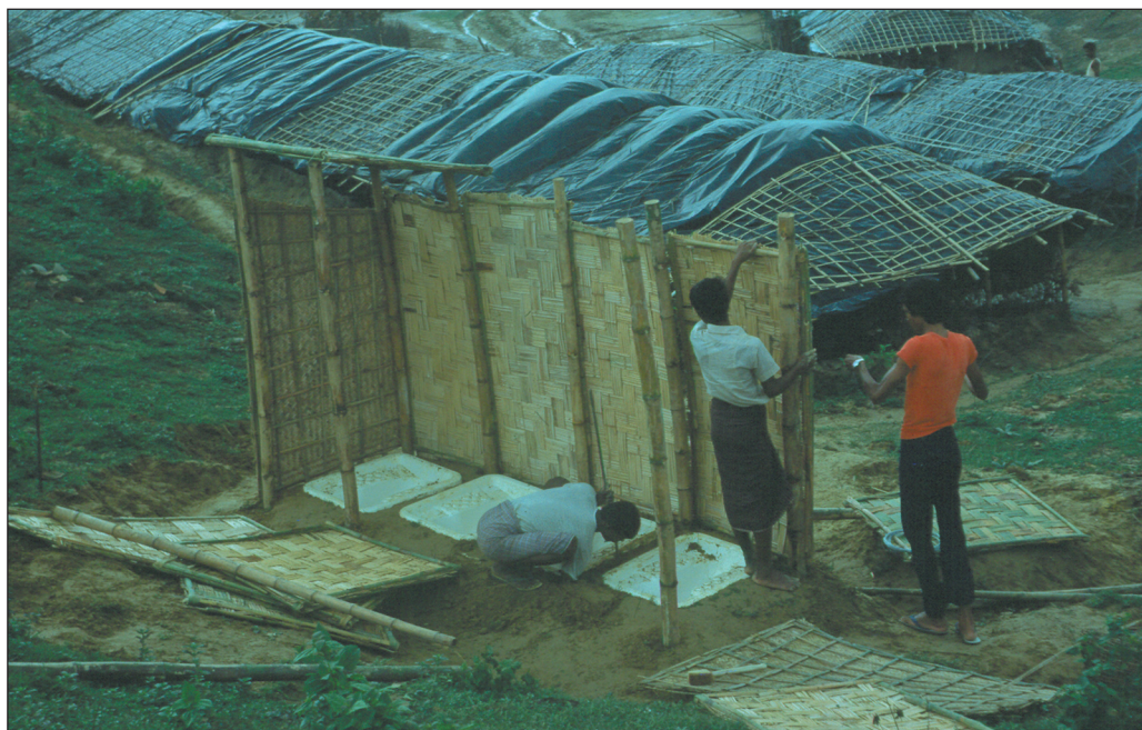
Borehole latrines nearing completion, Bangladesh
