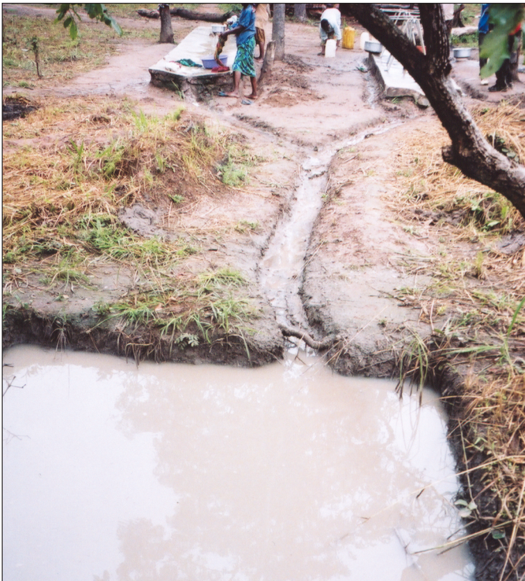
Poorly designed soakpit, Tanzania
