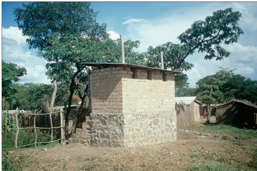
Raised VIP latrines, Tanzania
