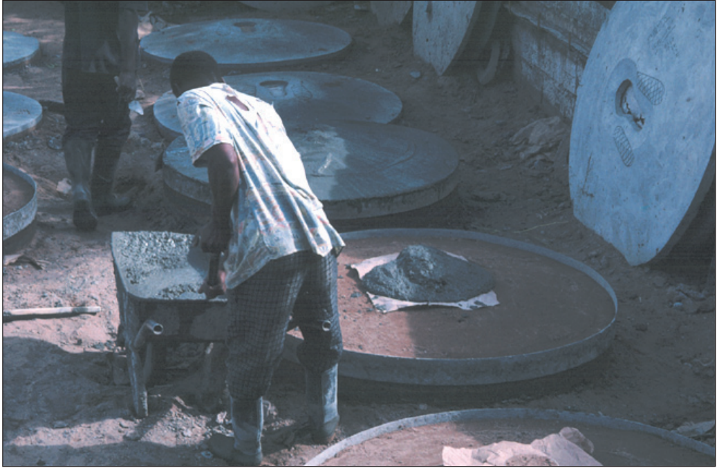
Producing latrine slabs in Mozambique
