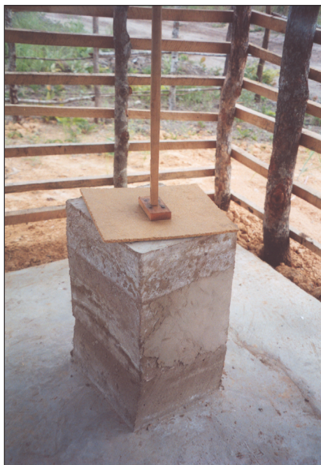
Sealed sharps pit, Zambia
