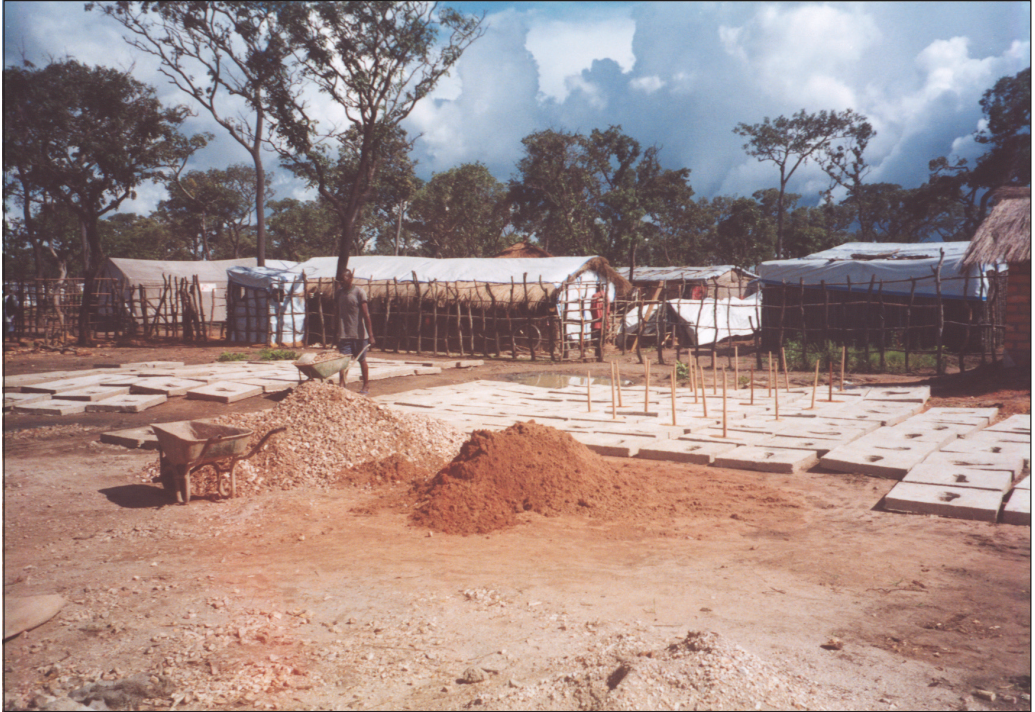
Preparation of concrete latrine slabs
