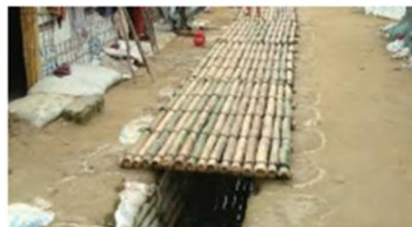
Covered channel in Cox's Bazar (IOM, 2018c).
