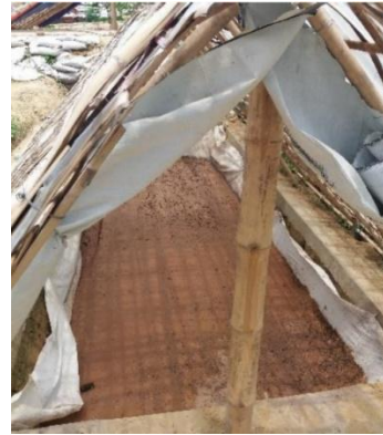
Infiltration bed (with roof protection against
