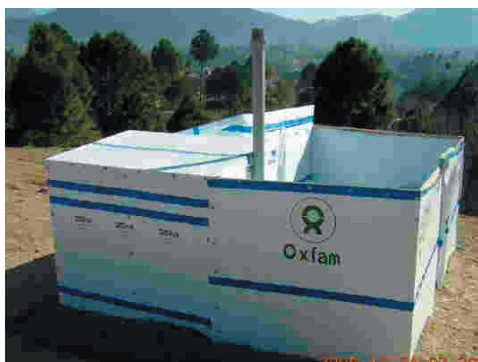
Photograph 1. Screened toilet and bathing unit
