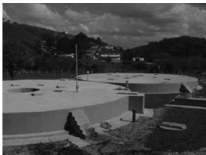
Figure 27.3. Anaerobic filter after upflow anaerobic sludge blanket (UASB) reactor (source: Colombo WWTP, SANEPAR/Brazil)
