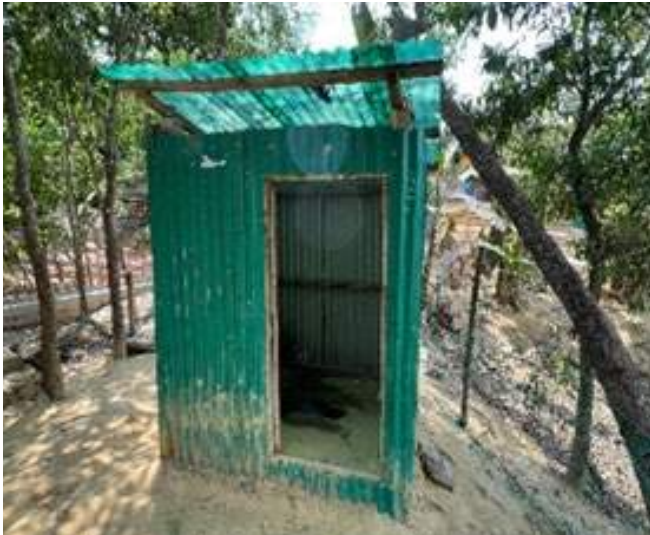
Figure 3: Direct pit single cubicle latrine example
