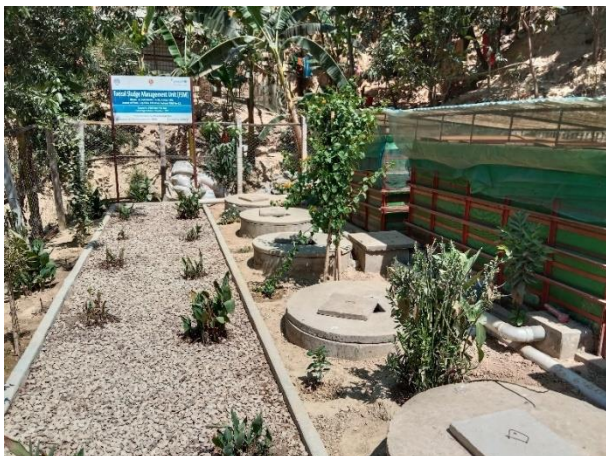
Planted filter and solids pits
