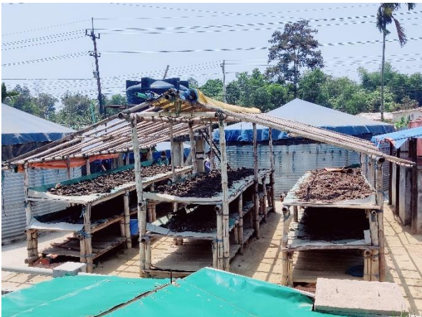
Solids drying and storage
