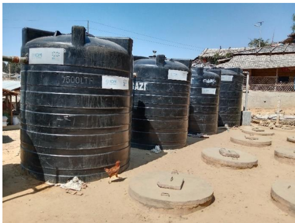
Biodigester and UFF tanks
