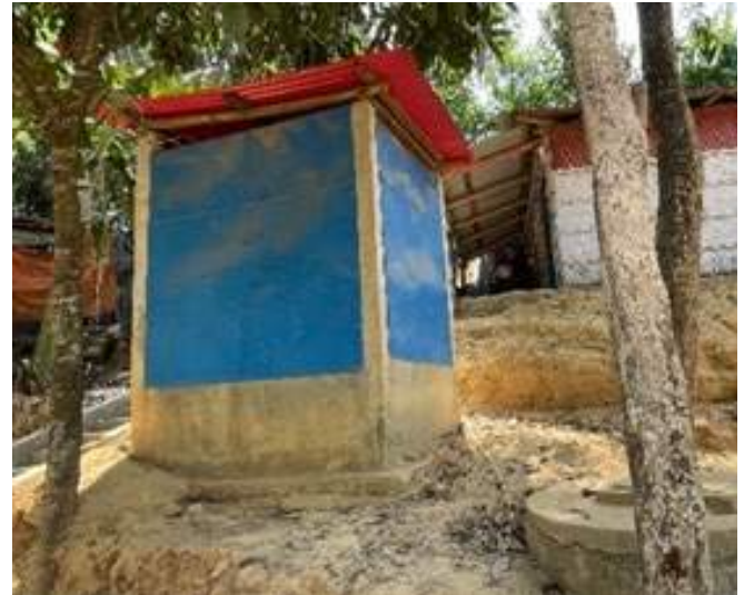
Figure 4: Direct pit with offset soak well single cubicle latrine example
