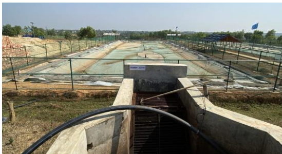
Anaerobic covered Lagoon
