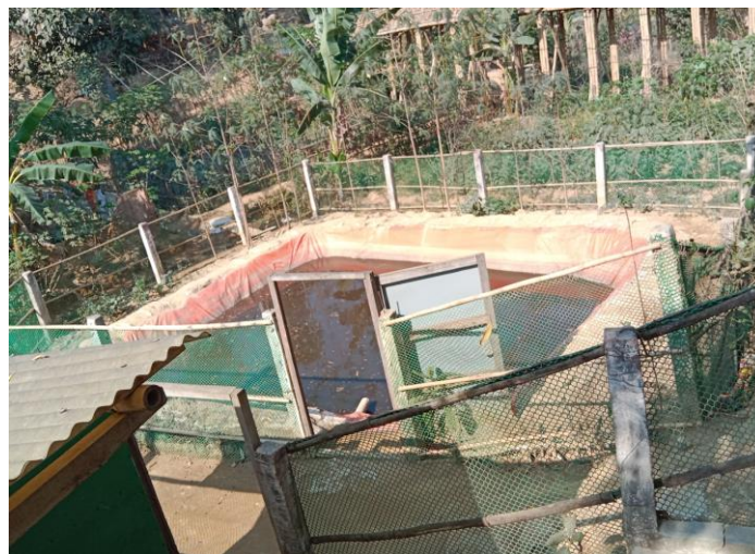
Photograph 1: Polishing Pond for one ABR site visited
