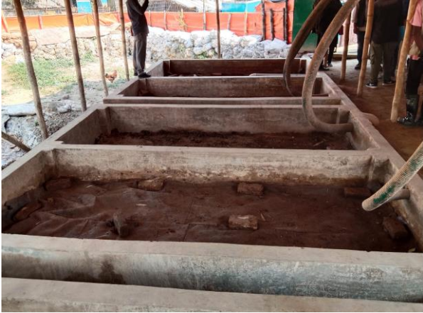
Drying and dewatering beds
