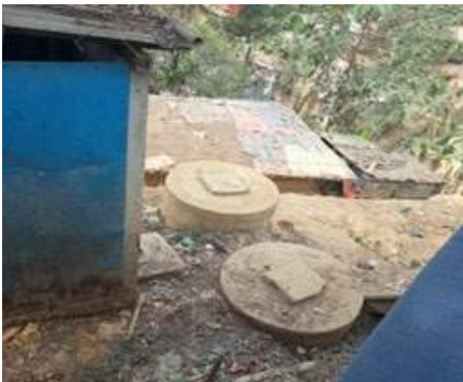
Figure 5: Twin pit offset single cubicle latrine example
