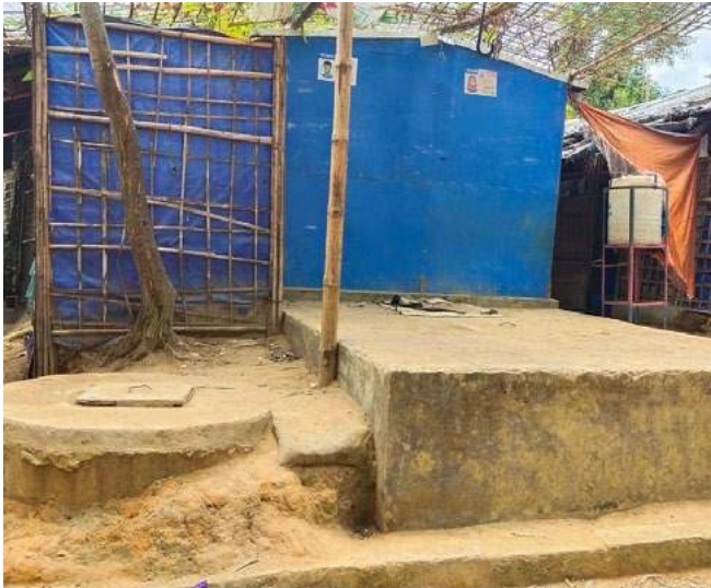
Figure 7: Septic tank with soak pit example
