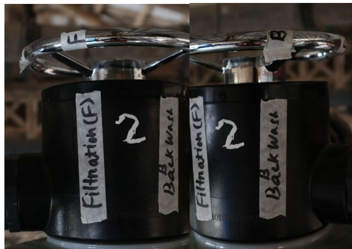
Pictures 13+14: Operation valve set on filtration or backwash
