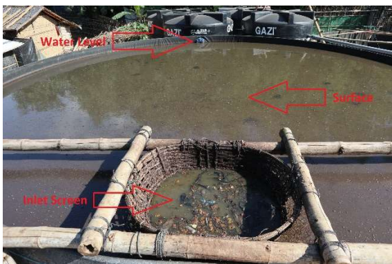
Picture 4: Screen, surface, water level
