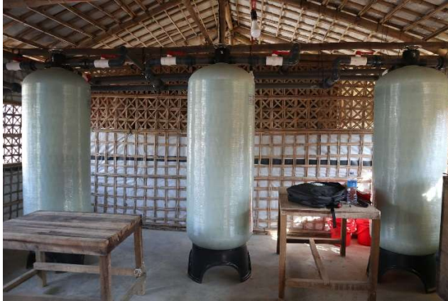
Picture 11: Glassbead filters
