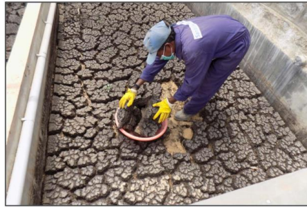
Figure 21: Removal of dry sludge
