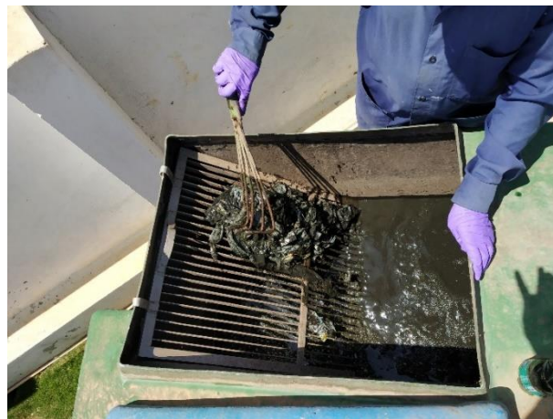
Figure 16 Removing solid waste from the screens with a trowel
