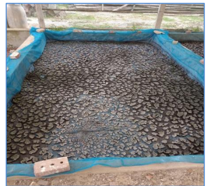
Figure 6: Existing Sludge Drying Bed
