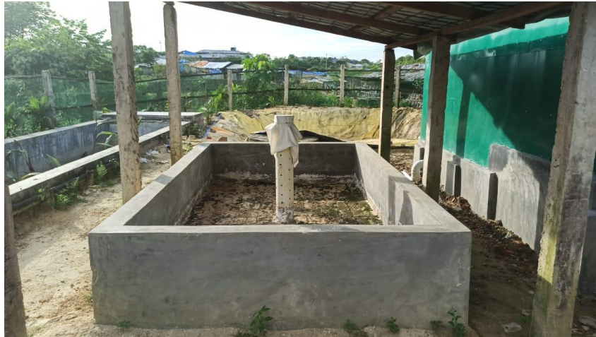
Picture: Drying Bed
