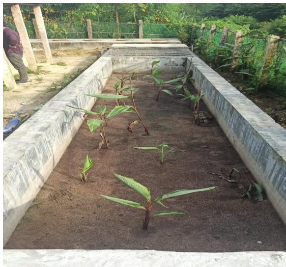
Picture: Planted gravel filter
