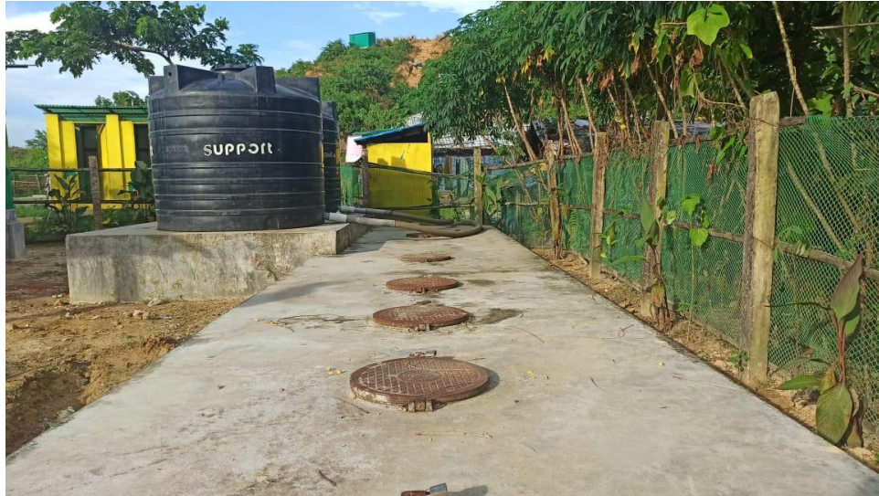
Figure: Anaerobic Baffle Reactor
