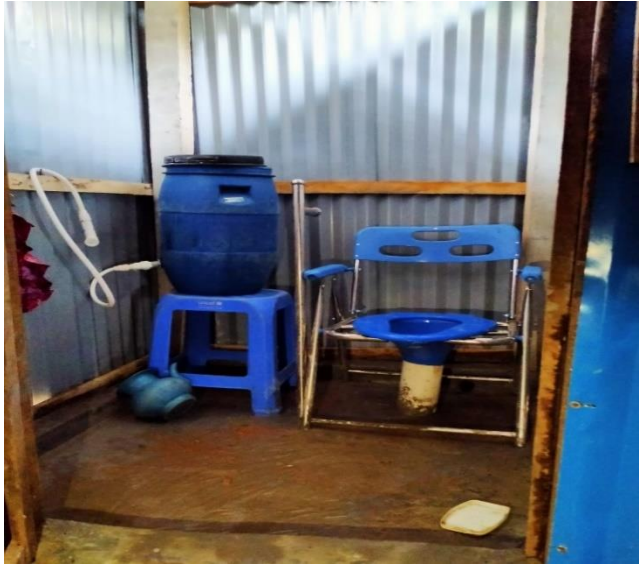
Picture 1: Persons with disabilities friendly latrines
