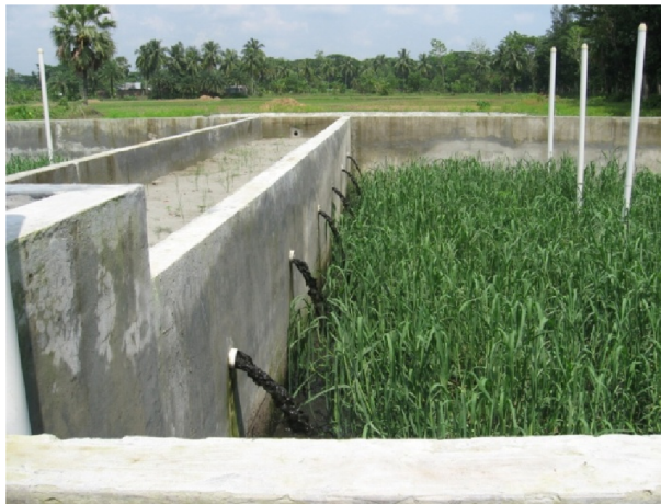
Figure-2b: Planted faecal sludge drying bed of FSTP at Lakshmipur Pourashava, Bangladesh
