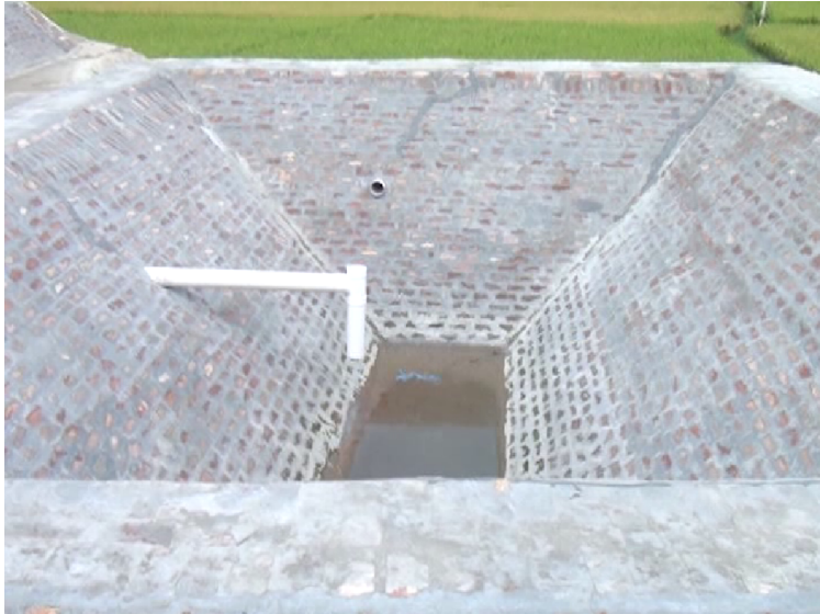
Figure-2c: Percolate collection pond of FSTP at Sirajganj Pourashava, Bangladesh
