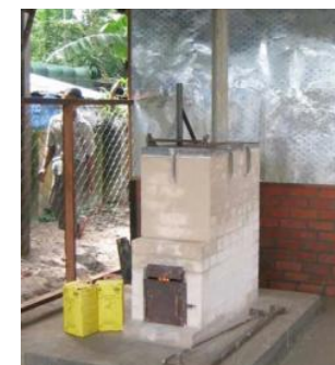
Example of De Montfort incinerator. (Source: PATH)
