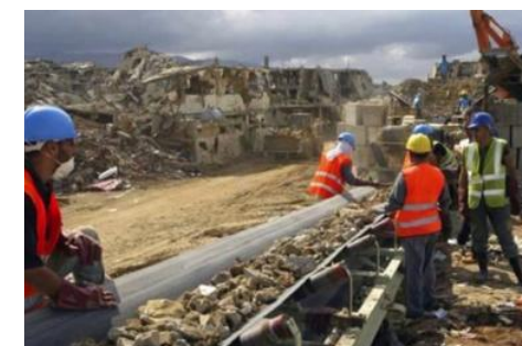
Example of community engagement for sorting and crushing of debris in Lebanon (Source: UNDP)
