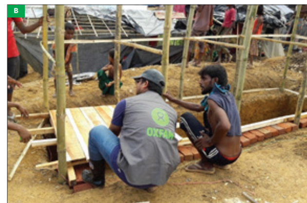
Figure 12: A Trench latrine in case of emergency (Courtesy: Oxfam).
