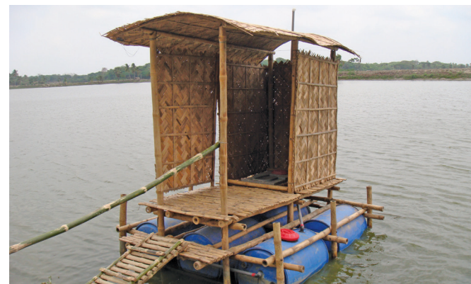
Figure 10: A floating latrine in haor area during flood (Courtesy: Oxfam)
