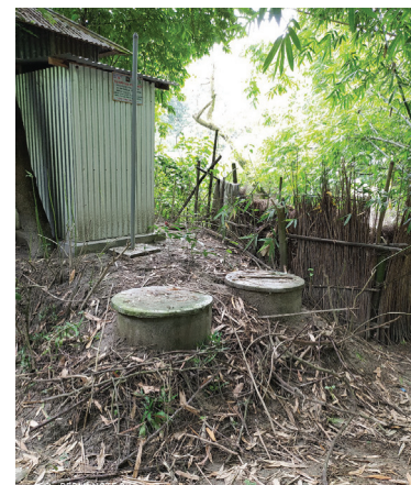
Figure 23: A raised offset twin pit latrine (Courtesy: Oxfam).
