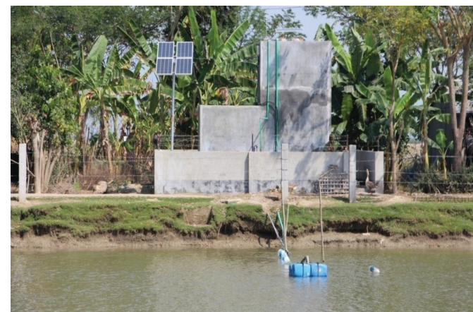
Figure 16: A solar powered pond sand filter (Courtesy: ITN-BUET)
