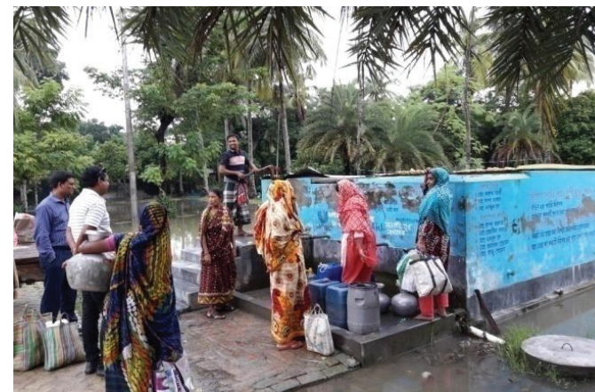
Figure 15: A normal pond sand filter (Courtesy: ITN-BUET)
