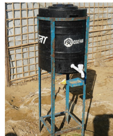
Figure 32: A 65-liter tank with tap and no handle over MS angle frame (Courtesy: Oxfam)
