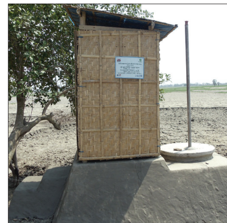
Figure 22: A raised offset single pit latrine (Courtesy: Oxfam)
