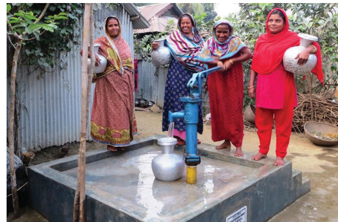
Figure 14: A deep-set tubewell in operation in a low groundwater level area (Courtesy: Concern Worldwide)
