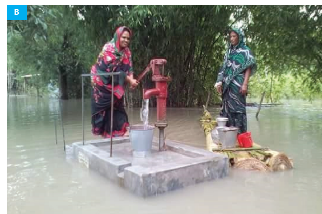
Figure 2: (A) Normal tubewell with raised platform (B) Raised platform with no. 6 handpump in use (Courtesy: Oxfam Bangladesh).
