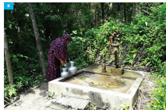
Figure 18: (A) Protected dug wells with tubewells to convey the water (B) Operational dug well in Assasuni, Satkhira (Courtesy: WaterAid and ITN-BUET).
