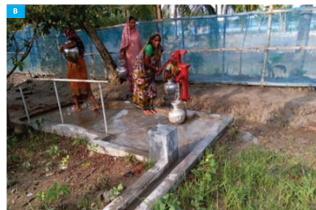
Figure 19: (A) Treated Pond for storing rainwater; (B) Users collecting stored water using a hand pump (Courtesy: Oxfam Bangladesh)
