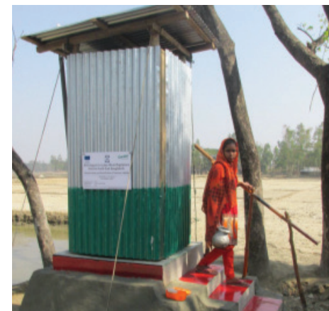
Figure 21: A raised direct single pit latrine installed in coastal areas (Courtesy: Concern Worldwide).
