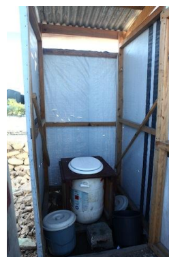
Photograph 4. Non-separating children's compost toilet
