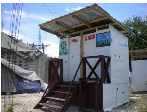
Photograph 1. SOIL UD Toilet, Jan 2011.
