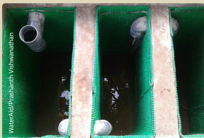
Figure 7: the bio-toilet’s three chambers
