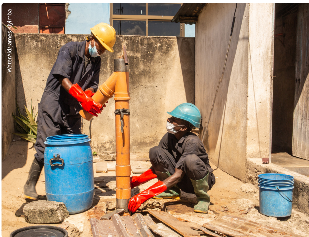
Figure 11: Sanitation workers in Dar es Salaam, Tanzania, operating a Gulper
