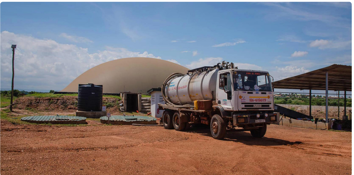
Figure 16: Safisana's biogas plant in Ashaiman, Ghana © Safisana
