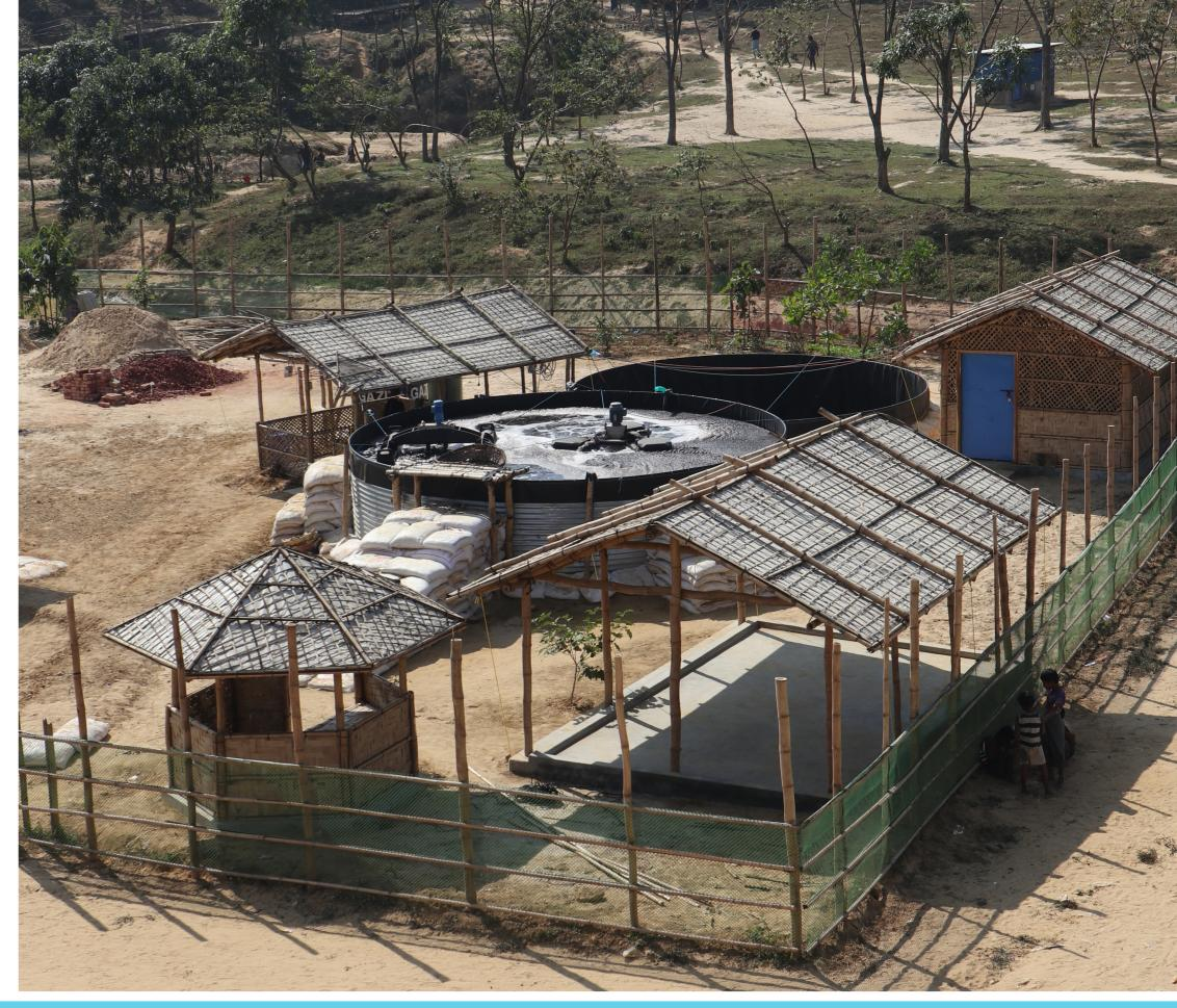
In 2018 IFRC piloted an aerobic waste treatment unit in the Bangladesh Population Movement Operation. Further improvements to the still operating system are being made and planning is underway for additional testing of a scaled up unit in other contexts. The treatment plant is accompanied by a faecal sludge field laboratory.
