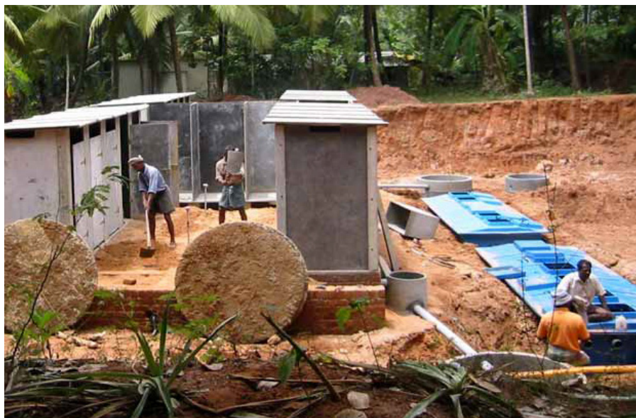
FIGURE 7: Construction of several toilet blocks connected to two pre-fabricated fiberglass ABR including a settling chamber, baffled reactor and an anaerobic filter unit (top). [9]
