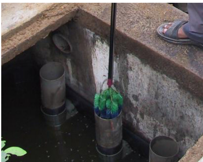
FIGURE 21: Cleaning the pipes with a brush (left) and desludging by vacuum truck (right). [25]
