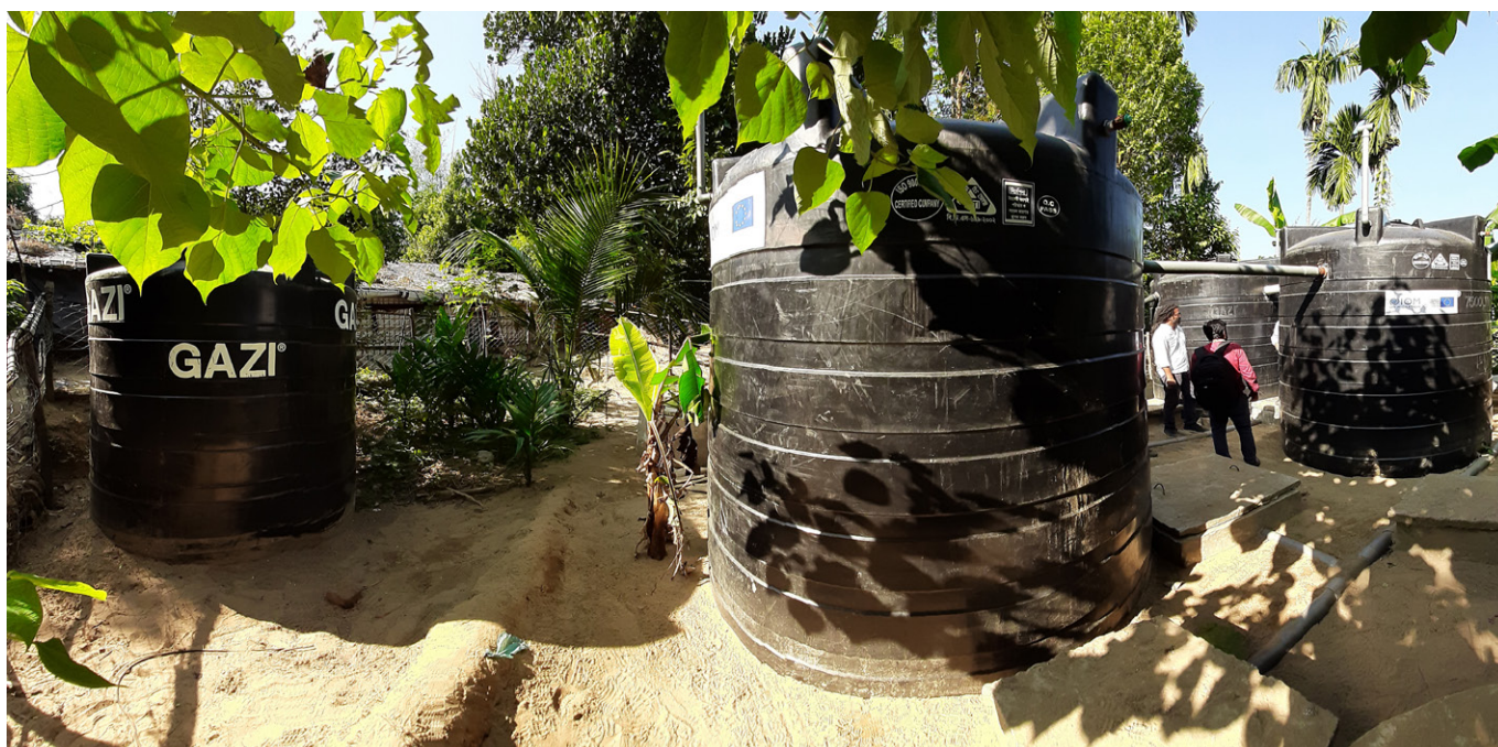
FIGURE 8: ABR and AF in rainwater harvesting plastic tanks installed Rohingya Refugee Camp 23, Bangladesh. [10]
