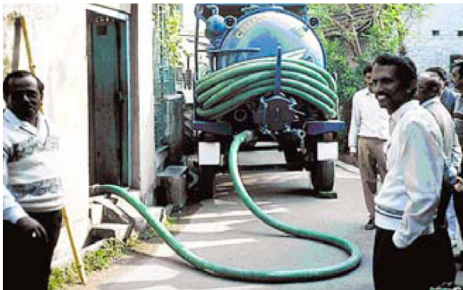
FIGURE 22: Desludging with vacuum pump and truck. [26]
