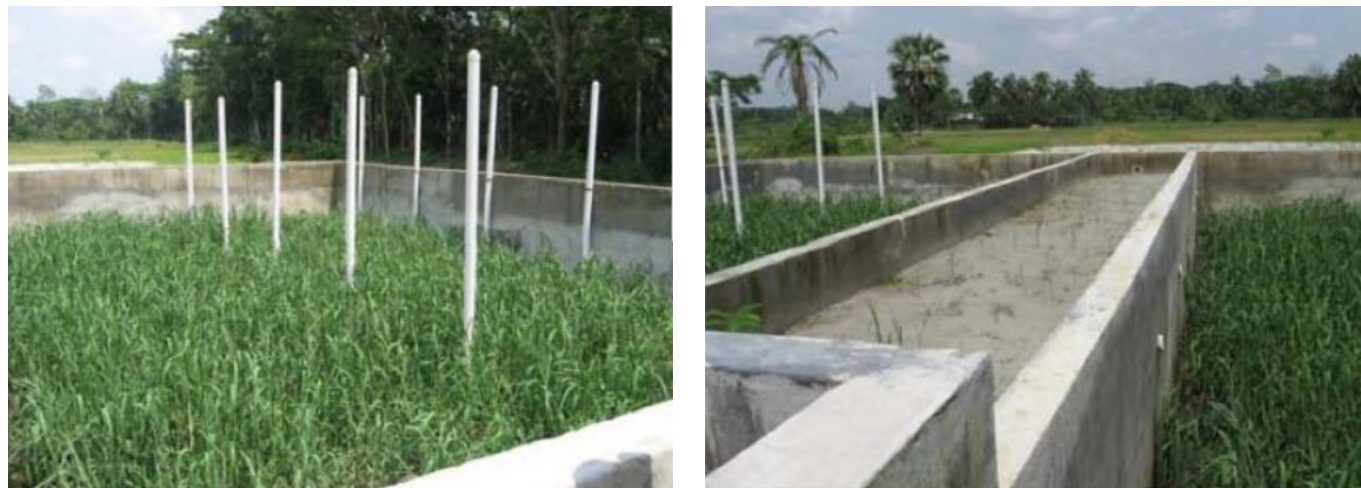
FIGURE 40: View on sludge drying beds in Lakshmipur, Bangladesh. [35]
