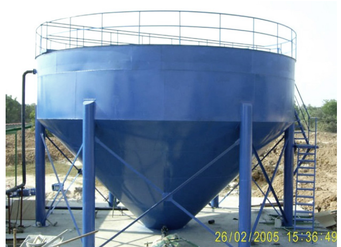
FIGURE 5: Cross-sectional view on a Gravity Settler (left) and one model constructed by Ashton Green & Company (right). [2]
