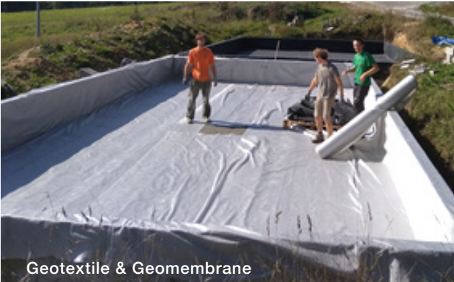
FIGURE 57: Liners and liner-passes for Horizontal filters.
