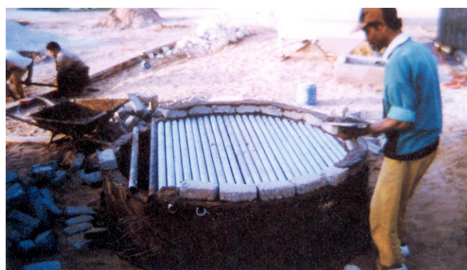
FIGURE 23: Test of a small sand filter as secondary treatment in a wastewater treatment plant, Ben Sergao, Morocco. [24]
