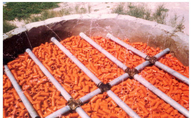
FIGURE 34: Plan and views of the drip body with secondary clarifier tested in Morocco. [32]
