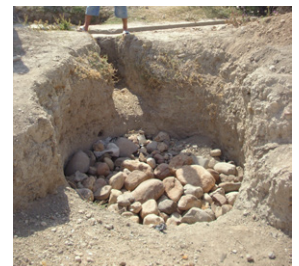
Soak Pit: high risk of contamination of groundwater
