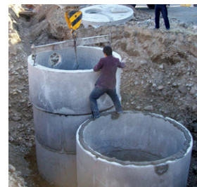
Soak Pit: high risk of contamination of groundwater
