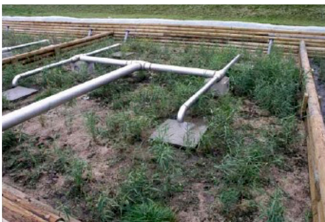
FIGURE 66: Feeding by aerial “H” system or overflowing pipes every 2 m. [59]
