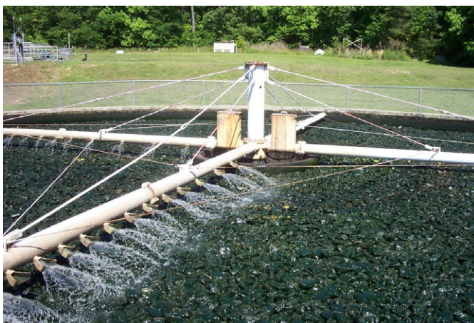
FIGURE 32: Rotating arms on a trickling filter (left) and fixed distribution pipes (right).
