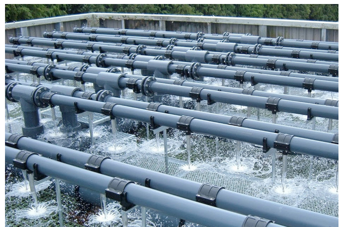
FIGURE 32: Rotating arms on a trickling filter (left) and fixed distribution pipes (right).
