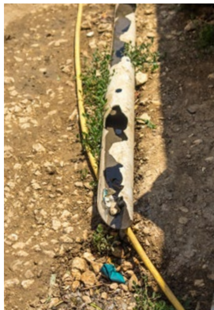
FIGURE 5: Shower drain without trap (left). Water pipe from the tank.
