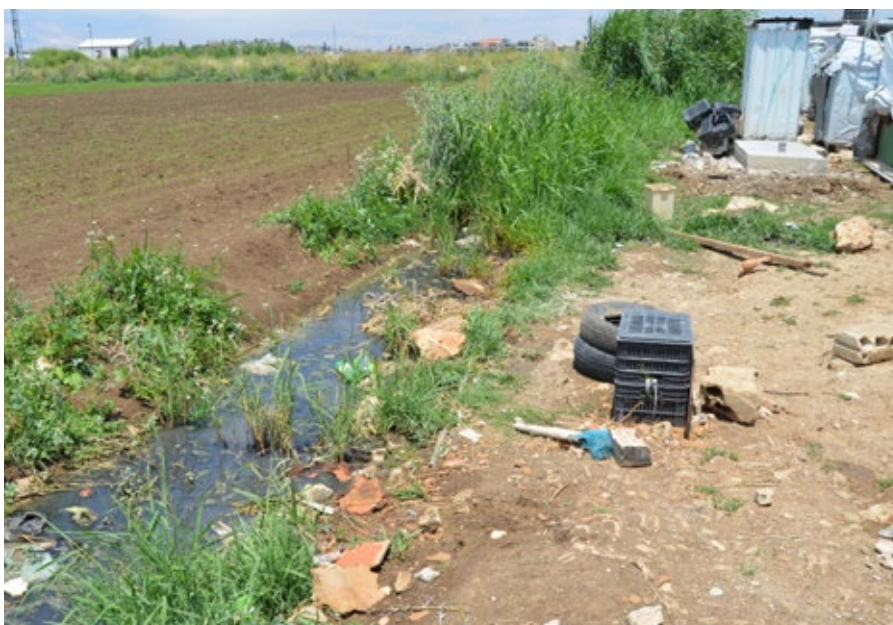
FIGURE 7: Stagnant water mainly from broken greywater pipes. The greywater is not treated, and it is freely discharged into the open drain.
