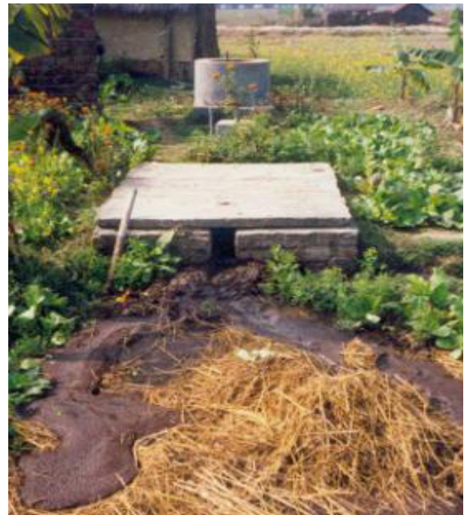
FIGURE 43: It is always better if the overflow of outlet is directly connected to the slurry pit and agriculture waste shall be put in this pit.
