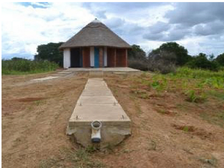
FIGURE 32: Biogas-toilet built on digester with well-sealed components.
