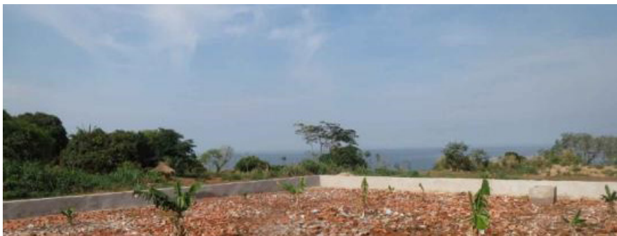
FIGURE 50: Banana planted in a gravel filter made of broken bricks.
