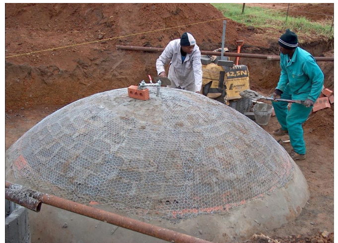
FIGURE 46: Finished digester with chicken wire in the outside plaster.
