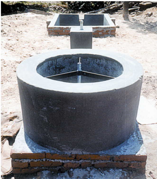
FIGURE 42: The axis of inlet, dome and outlet should be in 180°.
