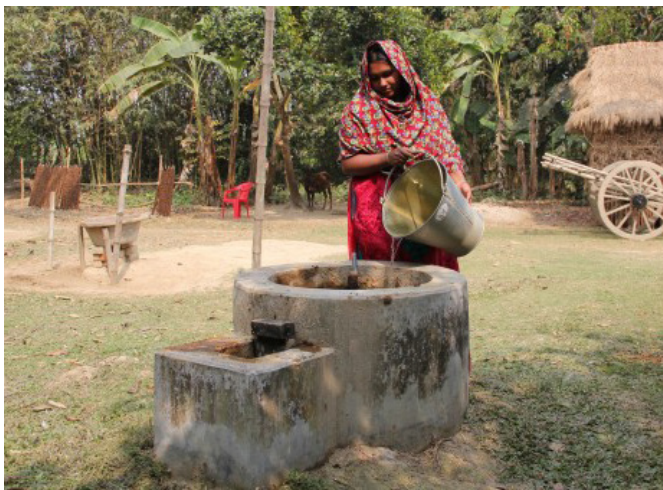
FIGURE 45: Feeding of the biogas plant: lifting of waste may not be convenient.
