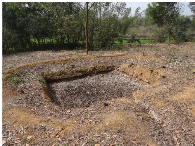
FIGURE 60: Open slurry pit in Balika, Mymensingh: Liquid leached and evaporated. The slurry is therefore completely dried out. The liquid effluent should be used as fertigation water.
