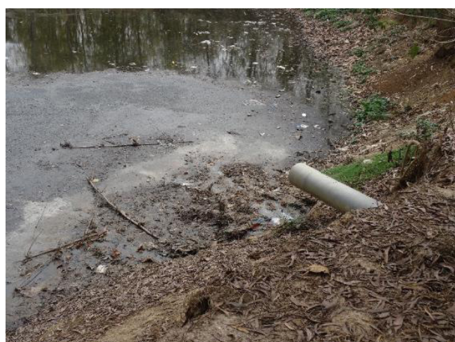
FIGURE 57: Poultry dropping based slurry; Slurry flows directly into the pond. Very poorly managed slurry pit of poultry-based biogas plant in Valuka, Mymensingh. This type of slurry pit will contaminate the surrounding and near water bodies.
