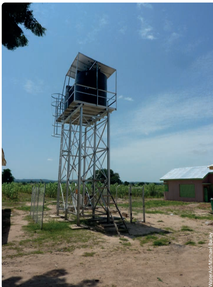
▲ Water storage tower with solar panels to power extraction pump, in Kafin Iya ward, Kirfi local government area, Bauchi state, Nigeria, September 2019.
