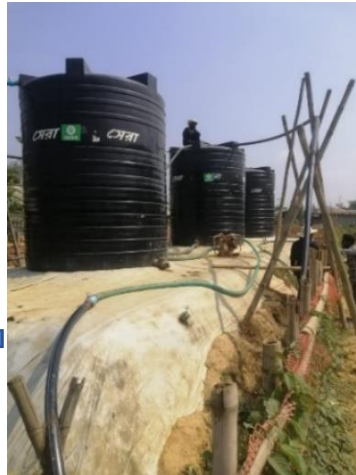
Figure 5: Pumping to NEXT TRANSFER station.
