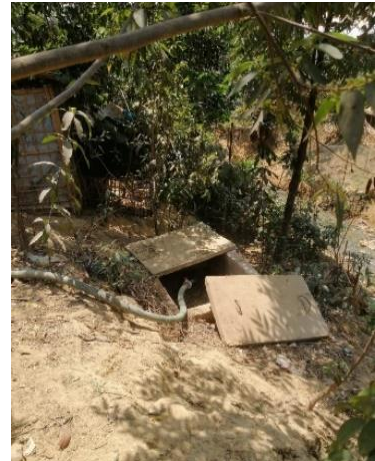
Figure 3: Transfer Pit/ Box / Transfer node
