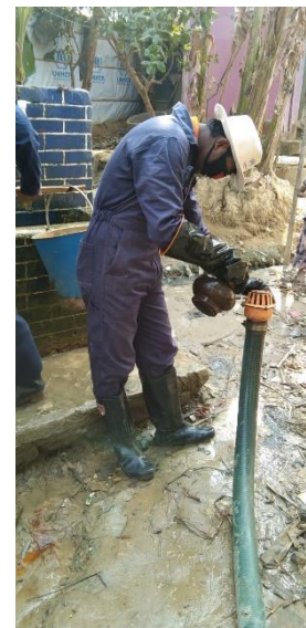
FIGURE 8: PRIMING OF ROBIN PUMP
