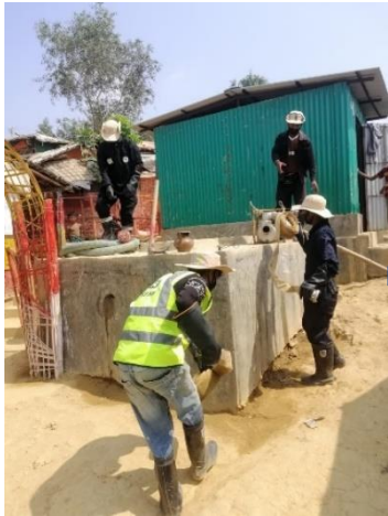
Figure 2: Desludging of latrines.
