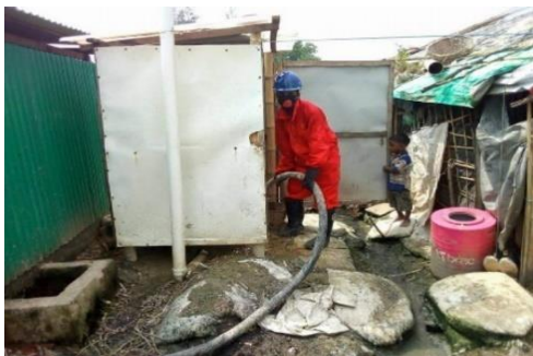
Figure 1: Emptying latrine containment
