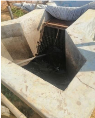
Figure 4: Pumped sludge received at FSTP intake.
