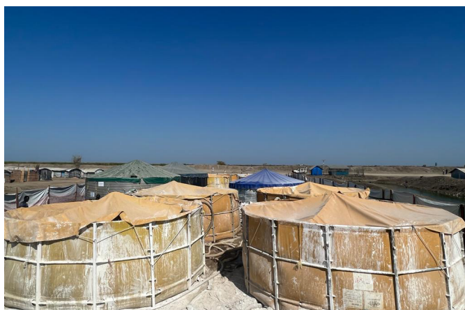
Figure 6: Different lime treatment tanks. Left: Metal frame tanks in Bentiu, South Sudan (source: IOM, 2023). Right: Treatment ponds constructed above-ground in Cox's Bazar, Bangladesh (source: Oxfam).
