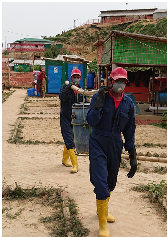
Figure 5: Emptiers carry a barrel of lime-treated sludge with a palanquin to the treatment plant in Cox's Bazar, Bangladesh (source: Eawag).
