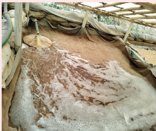
Photo: Unplanted drying bed.
