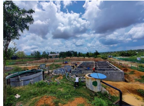
New Anaerobic Filter Reactor ( AFR), cross-section and image
