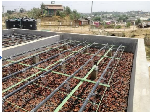
Trickling filter
