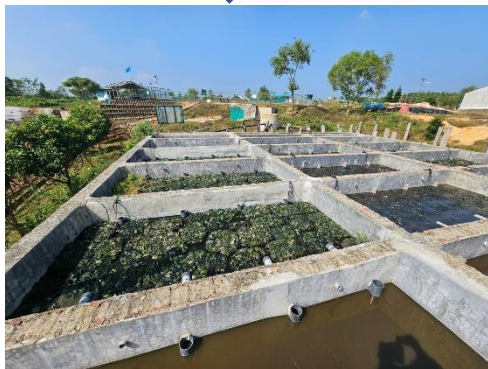
Anaerobic baffle and filter reactor
