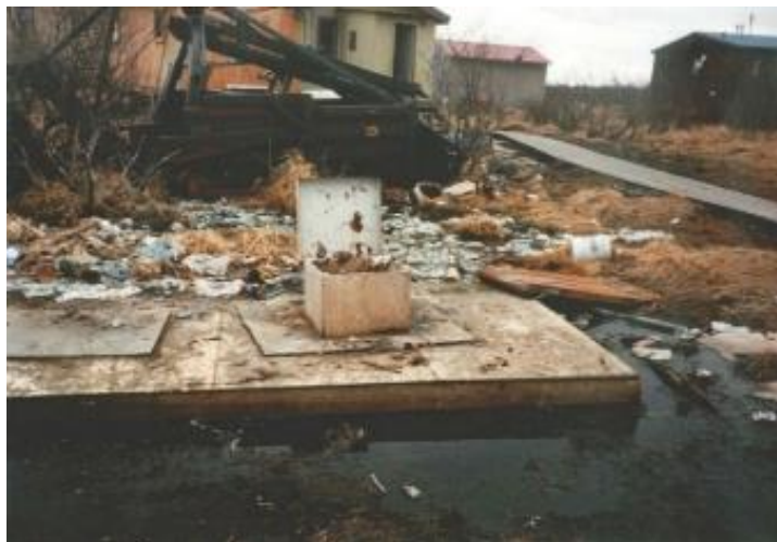
Photo A.1 Underground Communal Wastewater Tank, Alaska
