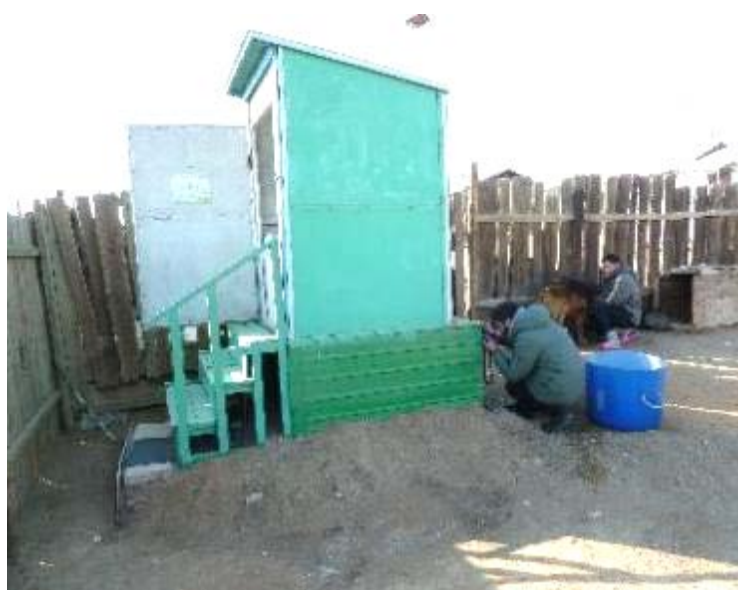
Photo 3.9 Container-Based Sanitation with Urine-Diverting Dry Latrine, Mongolia Source: World Bank.
