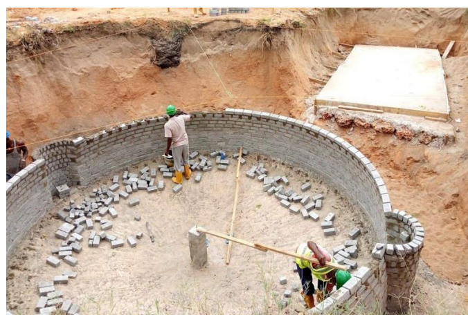
Bio-gas Digester construction
