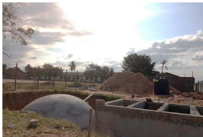
Anaerobic baffled reactor and Anaerobic filter construction
