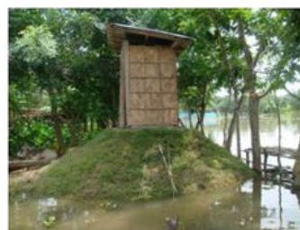
Earthen Raised Single Pit Latrine
