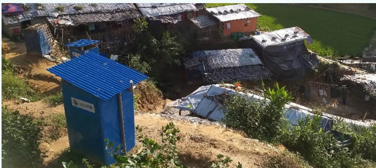
Figure 5: Emergency latrine in Cox’s Bazar, Bangladesh showing a large overhang. Solidarités International
