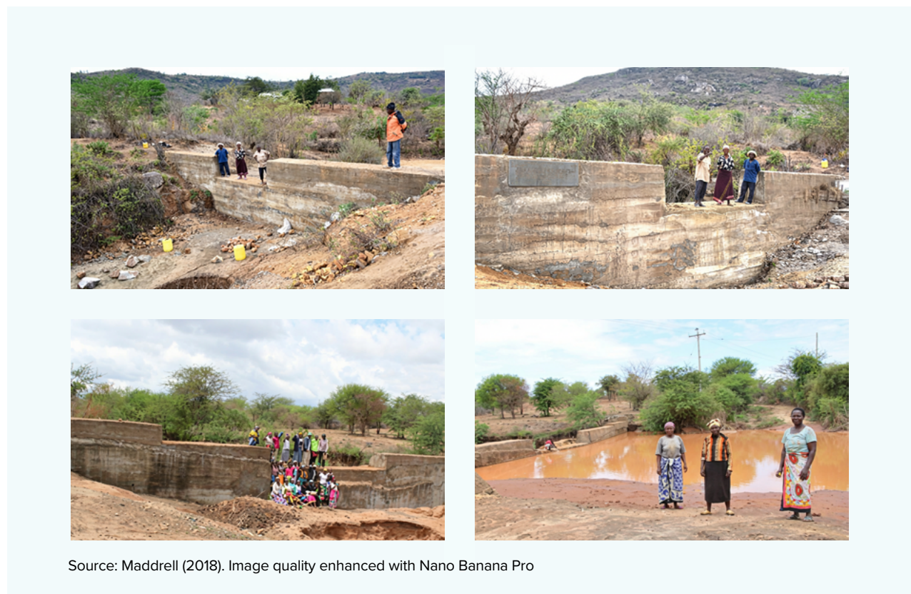
Figure 39: Photos of two sand dams to illustrate the different sizes: a 200 cement-bag sand dam (top) and a 850 cement-bag sand dam (bottom).
