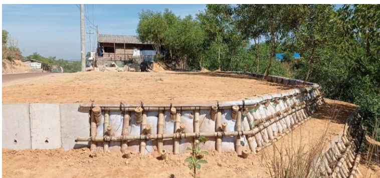
Figure 4: Site leveling and slope protection in Camp10.
